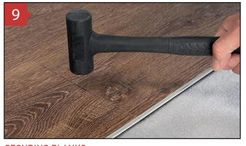
**SECURING PLANKS** As you go, don't forget to use a rubber mallet on the short sides to secure the locking.
