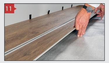
**DISASSEMBLING THE LONG SIDE** Lift up the entire row in the same angle as you did during installation, then slide the rows apart.
