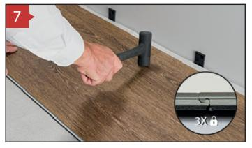
**ENGAGE 3**<sup>RD</sup> **PLANK ON SHORT SIDE (Part II)** Using a rubber mallet slightly tap the joints on the short side to secure. This ensures 3x locking.
